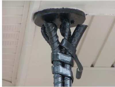
Completed Post & Railing
