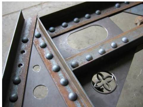
Roof Truss (Rivets!)
